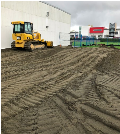
Tomsett Elementary – Installation of Pre-Load
