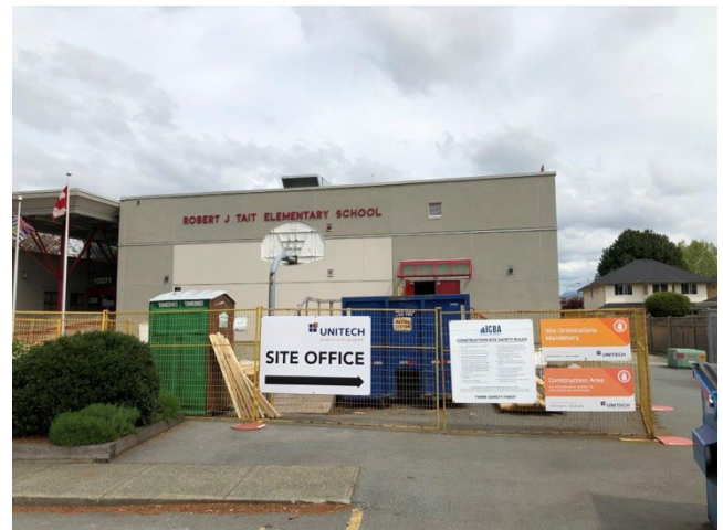
Tait Elementary – Front Entrance
